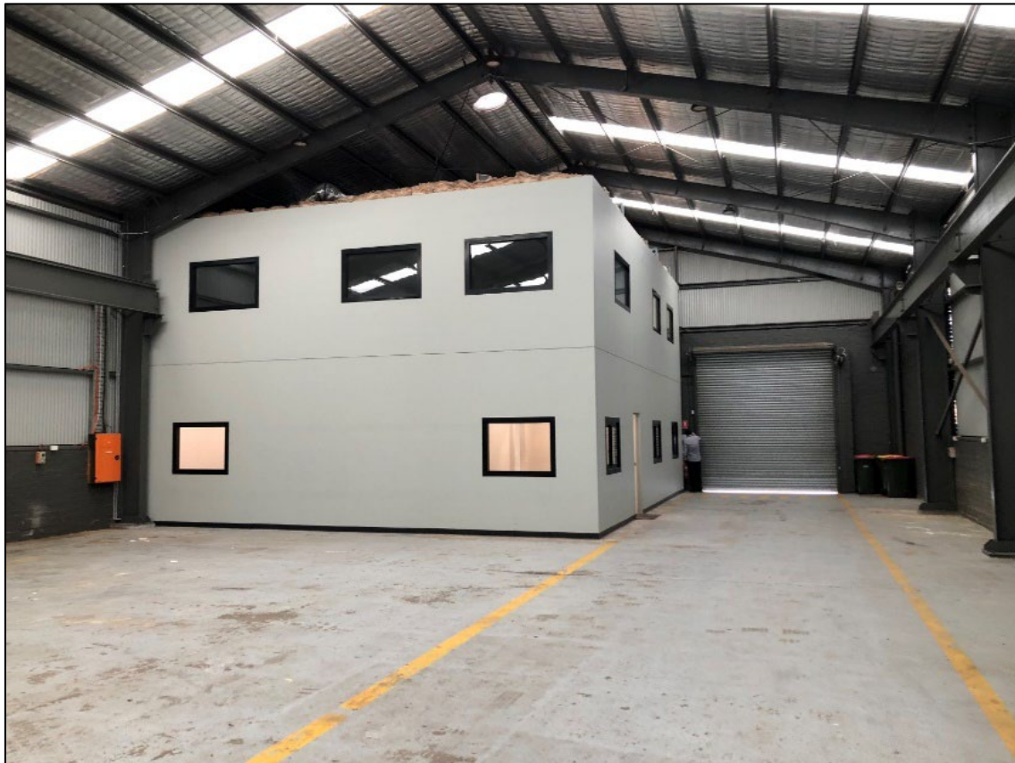
Figure 4: Internal warehouse and existing offices (Grose Street roller door in background) City of Parramatta Council, October 2024)
