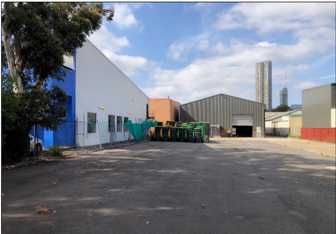
Figure 3: View from Fennel Street to the rear of the existing warehouse building (City of Parramatta Council, October 2024)
